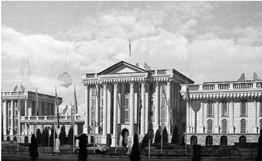
The old and the new Government Building
